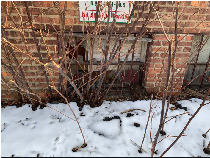
Figure 19: Broken windows and deteriorated brick at back of building.
