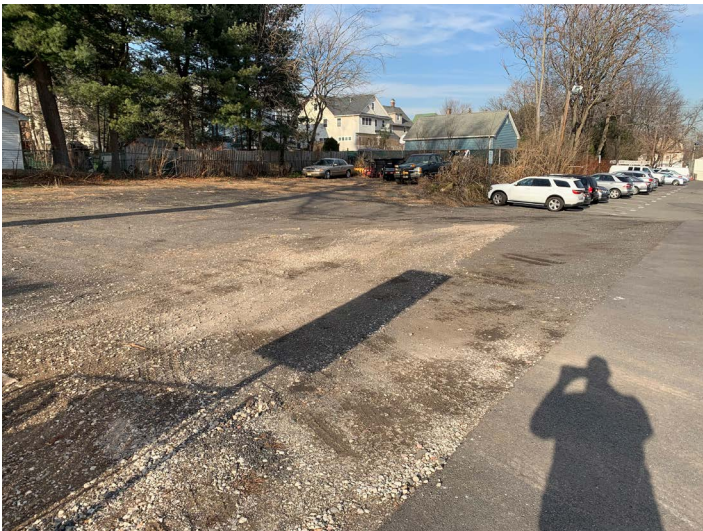
Figure 13: Deteriorated pavement in southwest corner of Lot 30.
