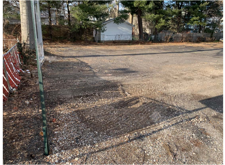
Figure 12: Deteriorated pavement in parking area on southwest corner of Lot 30.
