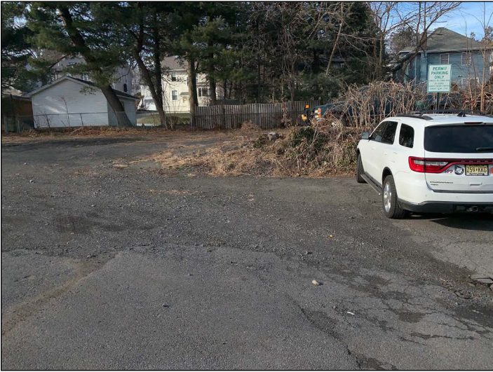
Figure 11: Grade change between parking / circulation areas on Lot 30 without barrier or striping.
