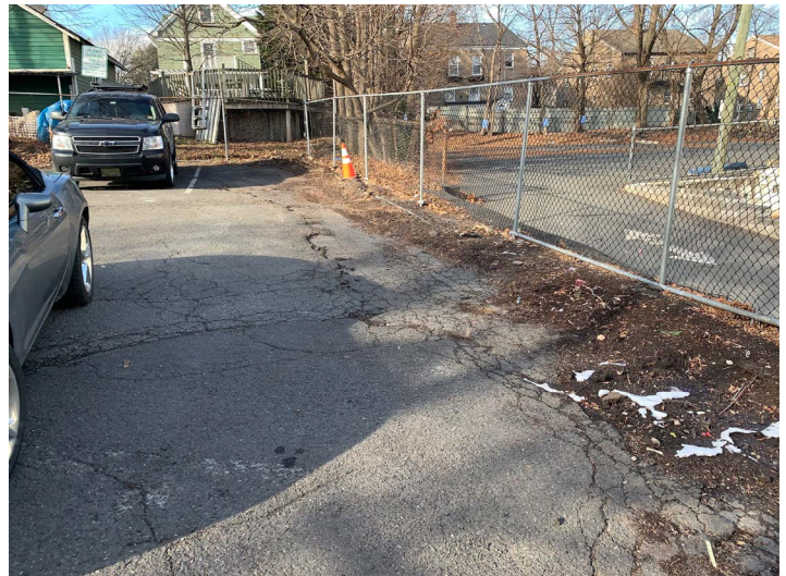
Figure 2: Deteriorated pavement in northwest corner of Lot 28.
