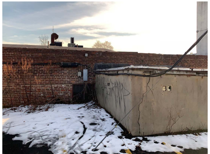
Figure 18: Deteriorated addition at rear of building.
