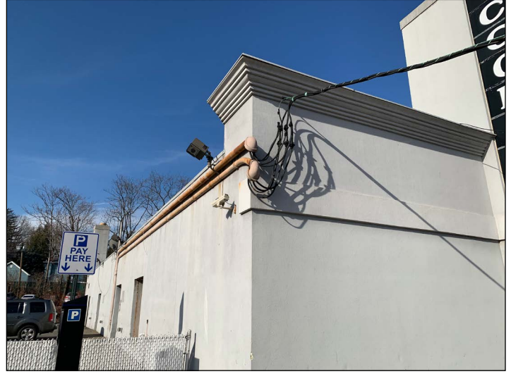
Figure 2: Electrical connection to building from street.
