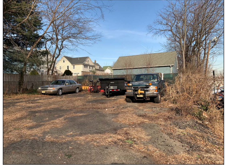
Figure 14: Deteriorated, overgrown parking area at southwest corner of Lot 30, with grade change to circulation aisle (right).
