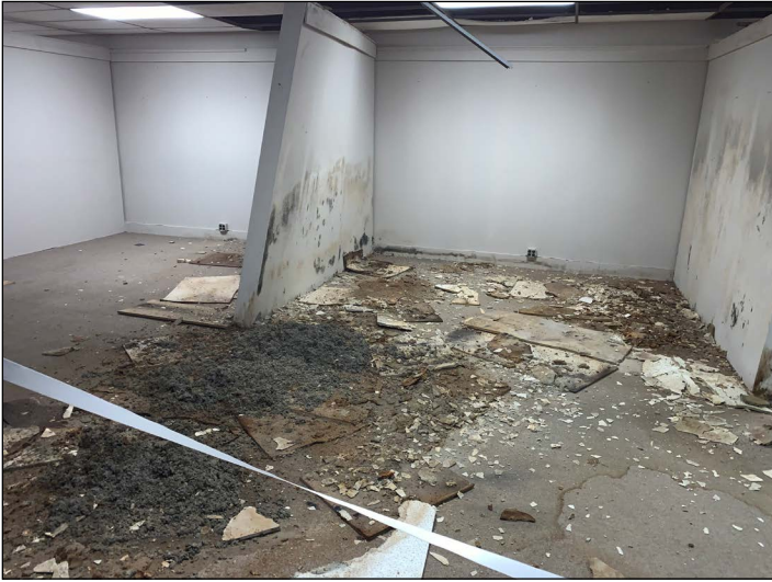
Figure 7: Debris and water damage from collapsed roof/ceiling.
