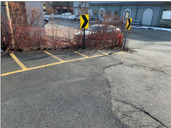
Figure 7: Grade change between Lot 28 and 29 without protective barrier.
