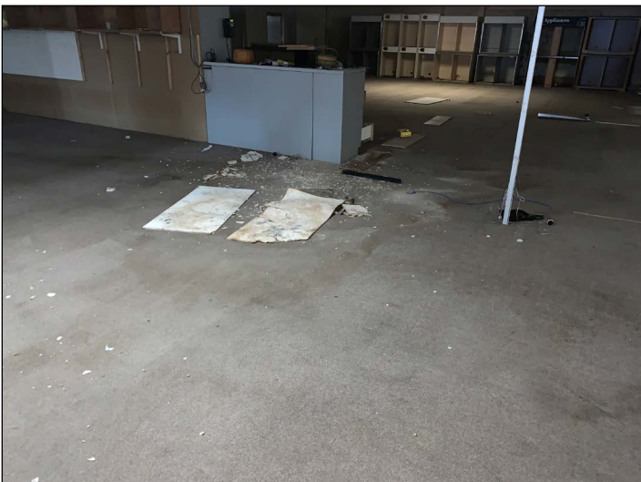
Figure 9: Debris from fallen, water damaged ceiling panels.
