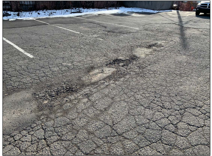
Figure 6: Deteriorated pavement in access aisle on Lot 28
