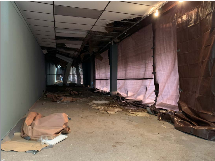
Figure 3: Section of interior with collapsing ceiling, debris, and water damage.
