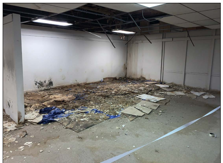
Figure 6: Debris and water damage from collapsed roof/ceiling
