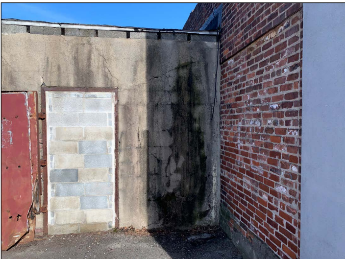
Figure 17: Wall damage with water staining on rear addition to building. Door opening shut with bricks, and old door loosely attached.
