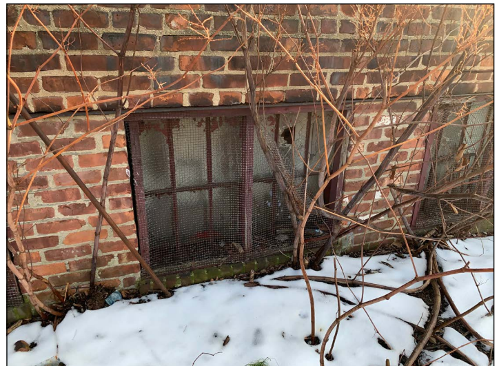
Figure 20: Broken windows and deteriorated brick at back of building.
