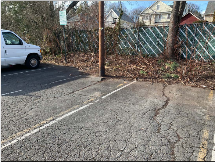
Figure 5: Deteriorated pavement on Lot 28, and utility pole at front end of a delineated parking space
